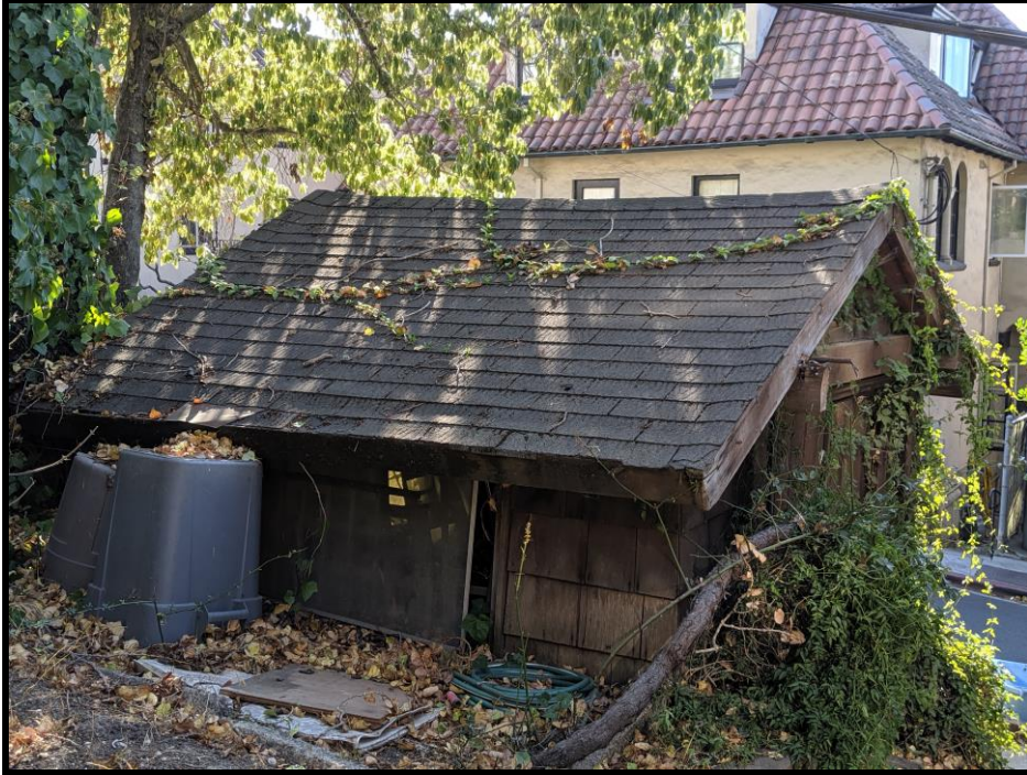
Figure 11: 1 Panoramic Way - accessory structure (playhouse), east façade
