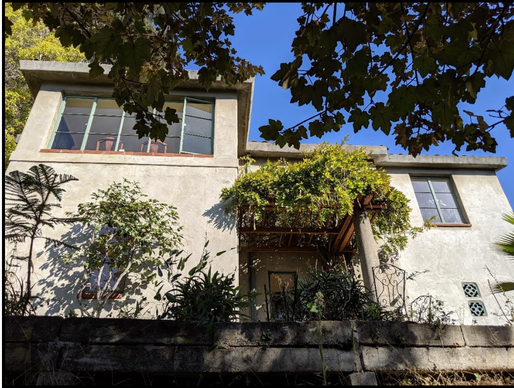
Figure 27: 4 Mosswood Lane - rear (west) facade
