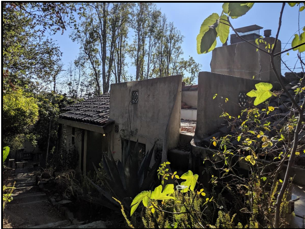
Figure 14: 4 Mosswood Lane - primary (east) facade, facing south
