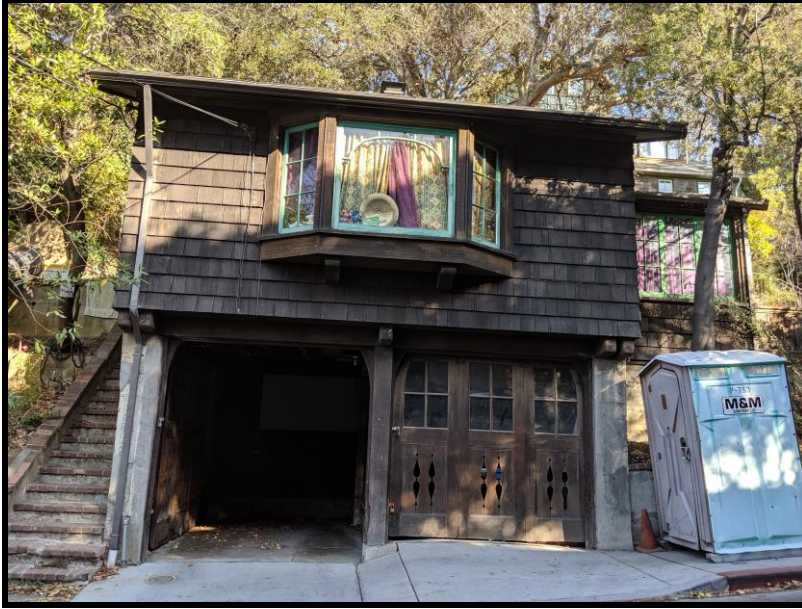
Figure 1: 1 Panoramic Way - one-story cottage atop two-car garage, primary (west) facade
