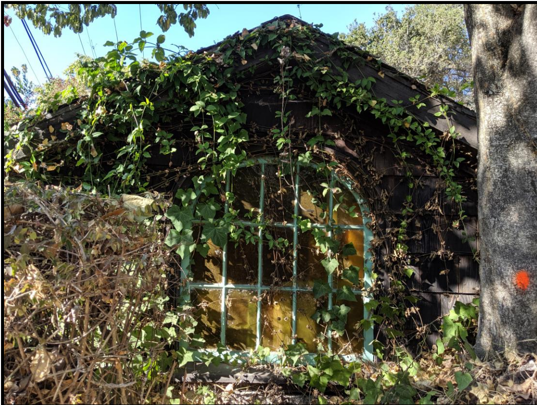
Figure 12: 1 Panoramic Way - accessory structure (playhouse), south façade
