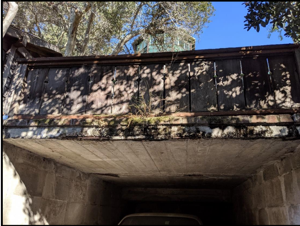
Figure 7: 1 Panoramic Way - carport with wood railing above
