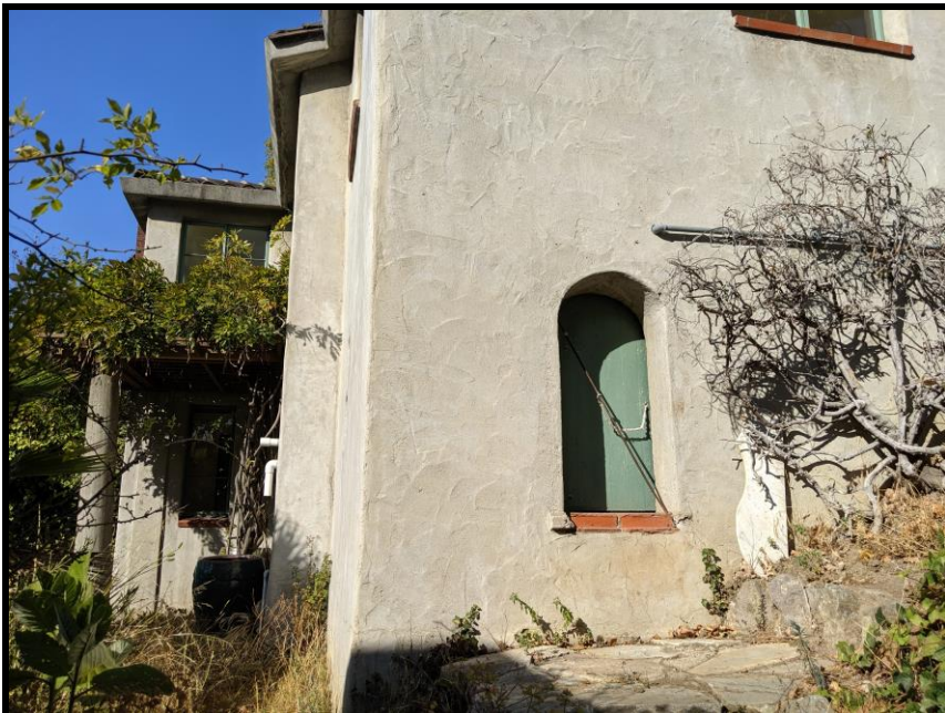
Figure 26: 4 Mosswood Lane - lower (west) portion of south facade
