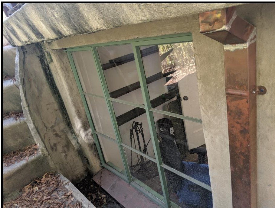
Figure 20: 4 Mosswood Lane - metal frame multi-lite window on east facade
