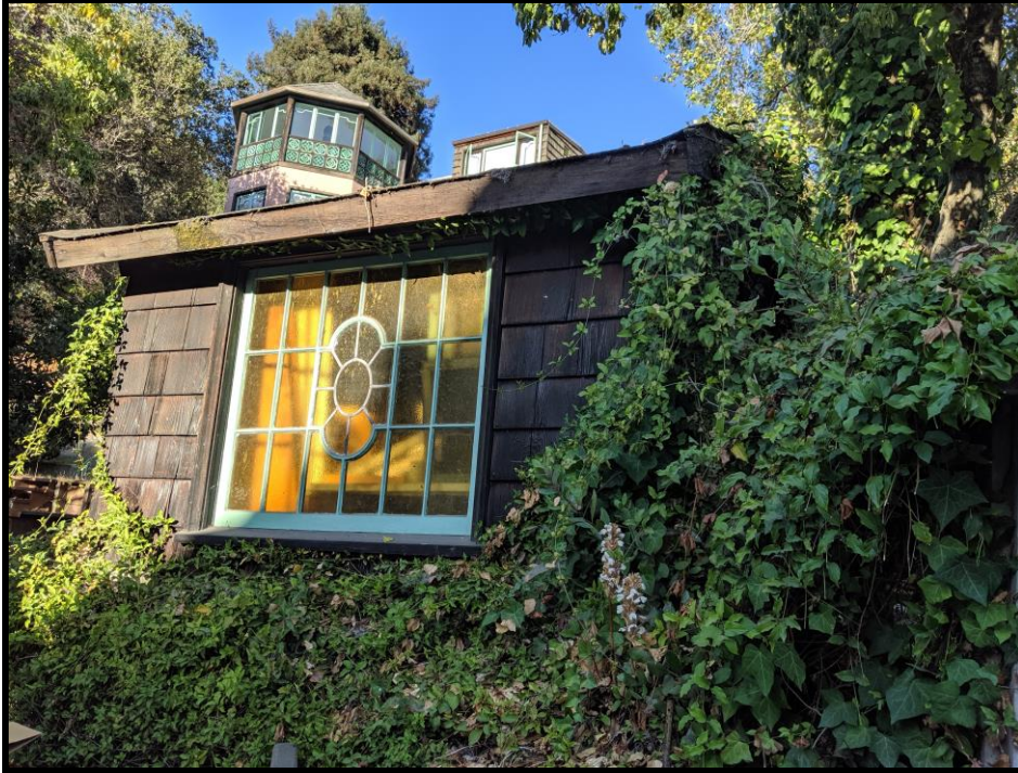
Figure 9: 1 Panoramic Way - accessory structure (playhouse), west façade
