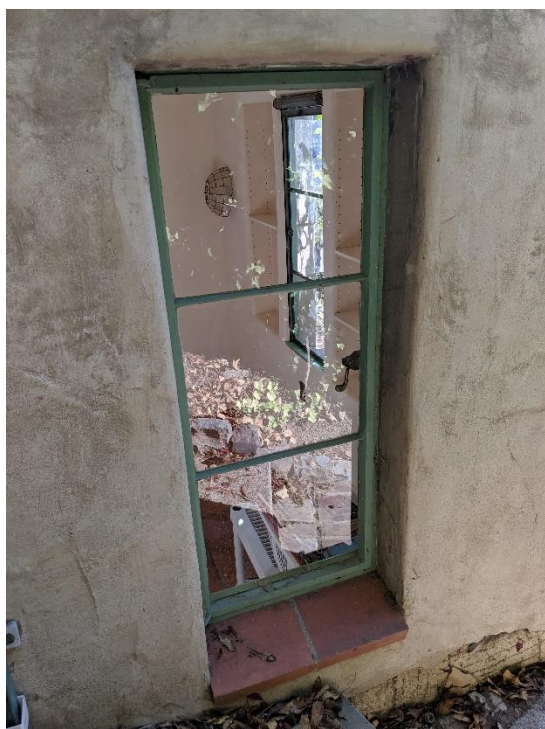
Figure 22: 4 Mosswood Lane - steel sash window with tile sill on north facade
