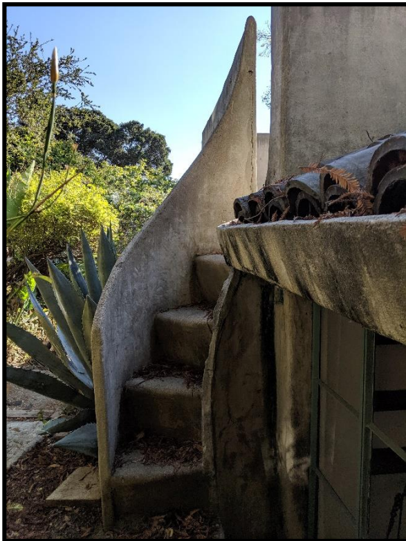
Figure 18: 4 Mosswood Lane - curving stairway on front (east) facade, facing south
