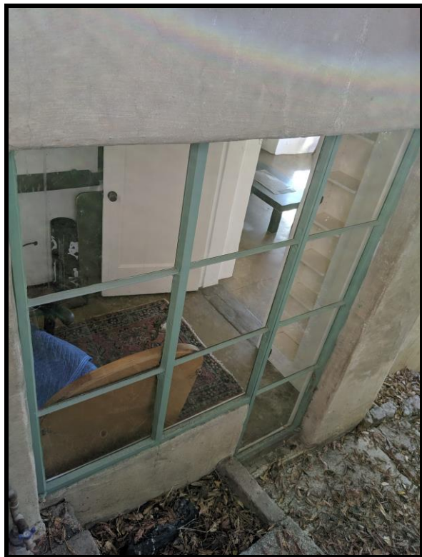
Figure 21: 4 Mosswood Lane - metal frame multi-lite window, north facade
