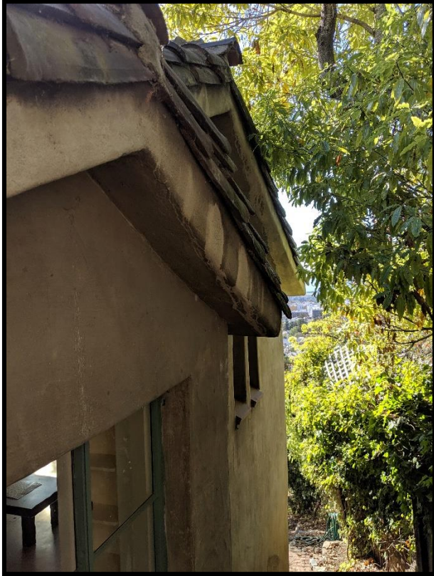
Figure 23: 4 Mosswood Lane - upper portion of north facade, facing west
