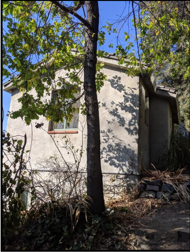
Figure 25: 4 Mosswood Lane – upper (east) portion of south facade
